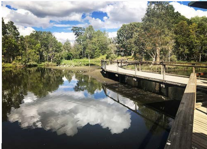
The Storm King® has been treating sewer overflows to the Bowies Flat Wetland in Brisbane for more than 15 years ©Hydro International
