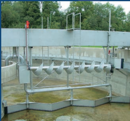
„with suction scrapers and effluent troughs“
