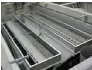
The clarified water collected in the V-notch weirs is transported to the outlet flume
