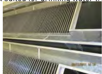
The clarified water collected in the V-notch weirs is transported to the outlet flume
