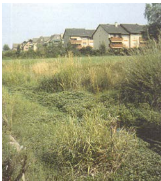
The same point after installation of a ROMAG CSO screen (CSO = Combined Sewer Overflow)
