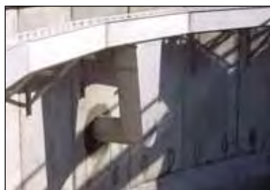
KD 16.18 stainless steel channel with outlet.
