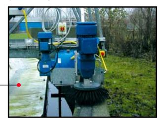
The runway brush consists of a gear motor and a nylon brush that that is mounted on a bracket. Through the rigging screw the height is adjusted, so nylon brush are constantly in contact with the runway brush.
