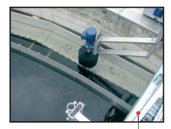
The channel brush model KD16.11 is meant for use in e.g. settling tanks in which it cleans the sides and bottom of the effluent channel as well as the sides of the overflow weir. The suspension bracket makes it very easy to attach the brush to any peripherally driven scraper bridge model KD 16.
