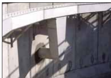
KD 16.18 stainless steel channel with outlet.
