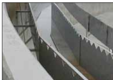
KD 16.18 stainless steel channel with V-notch weir on both sides, as well as KD 16.17 scum board.
