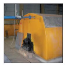
The FSM Center Flow Screen was developed to deal with particular problems associated with waste water pre-treatment and raw water intake.
