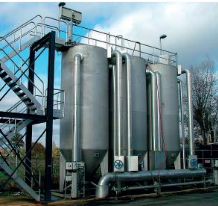
Installation of DynaSand filters in WWP Bree, Belgium.
