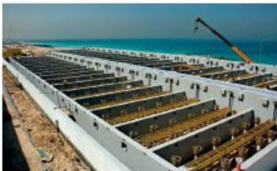
Desalination plant in Dubai based on DynaSand sand filters.
