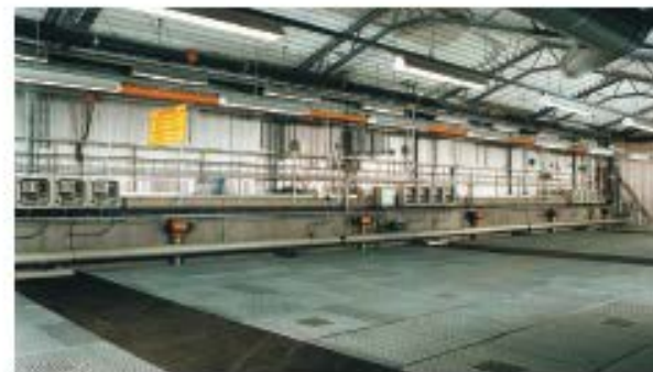
Filter basin covered with flooring.
