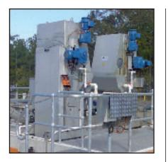
The FSM Dual Flow Screen was developed to deal with particular problems associated with waste water pre-treatment and raw water intake.
