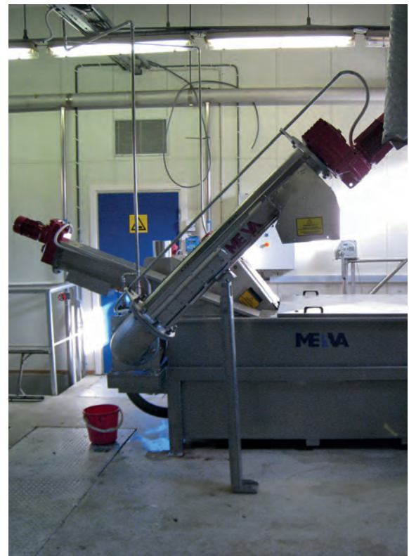
Meva SRS with a grit screw. Screen connected to SWP and CPS.
